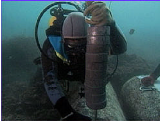
Diver attaching lead line.
